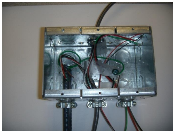
Fig. 3-4 Rough Plumbing and Wiring to Rough-in box, Flush Mount Unit
